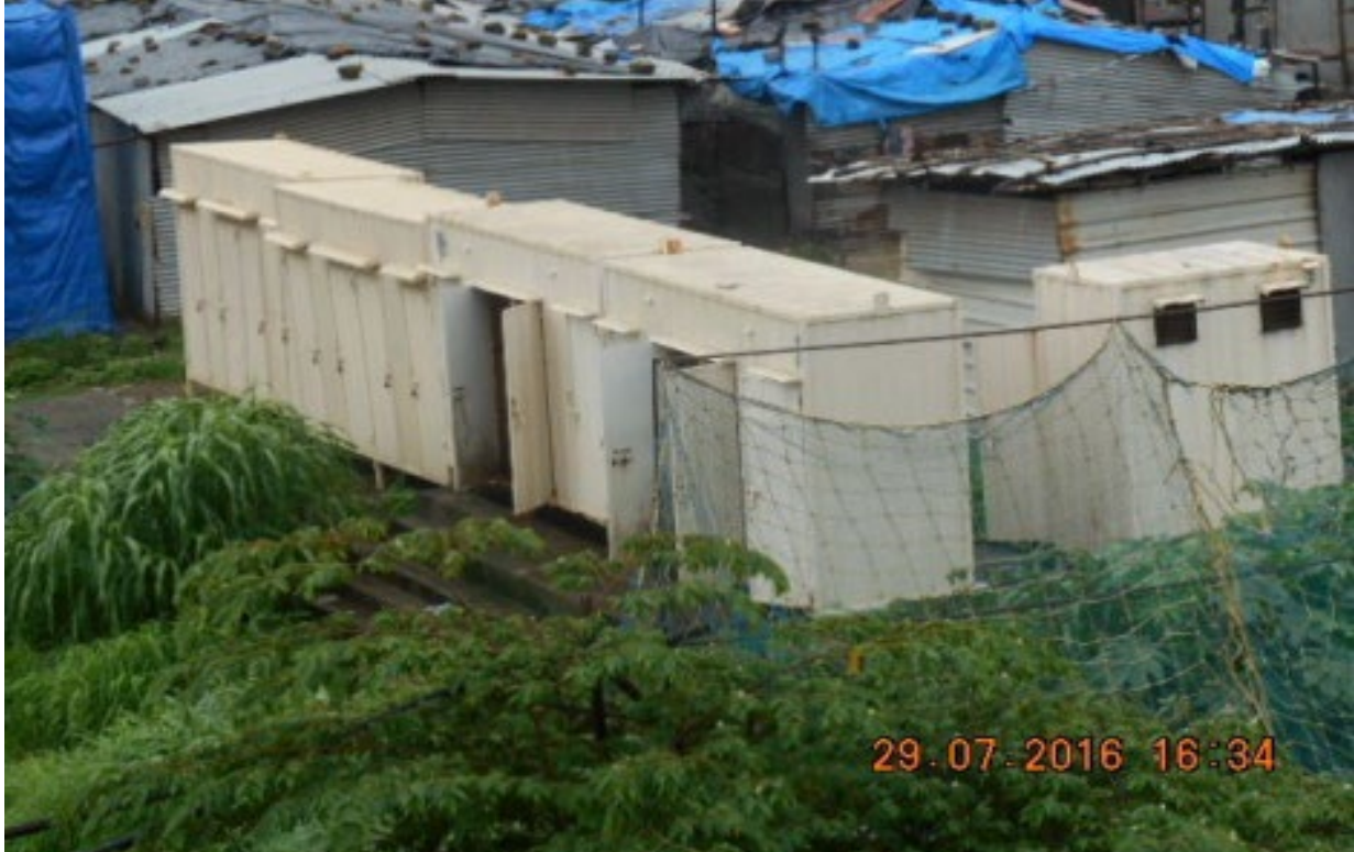
Toilets for Labour
